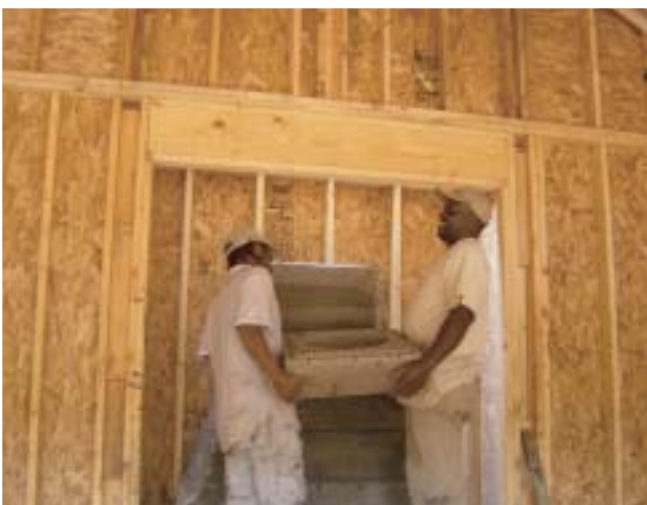
Step 5 · Set Chimney Blocks in place
