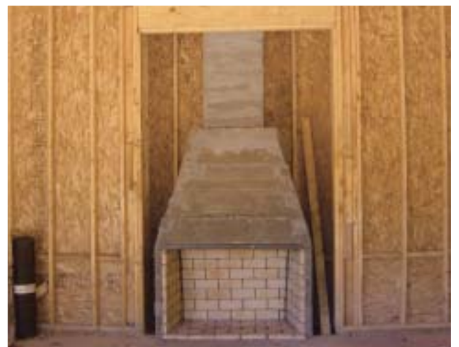
Step 6 · Install Firebrick and fireplace is complete
