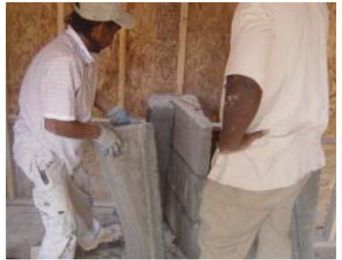
Step 2 · Fire Box Sides set, start building the back
