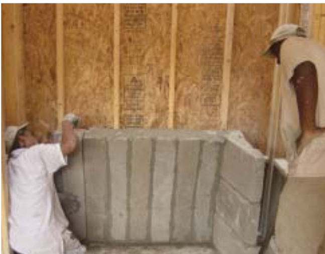
Step 3 · Place Centerbacks along rear of Base Plate
