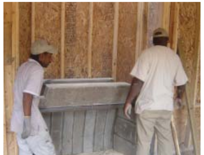
Step 4 · Set High-Draft Throat along top/ build Smoke Chamber
